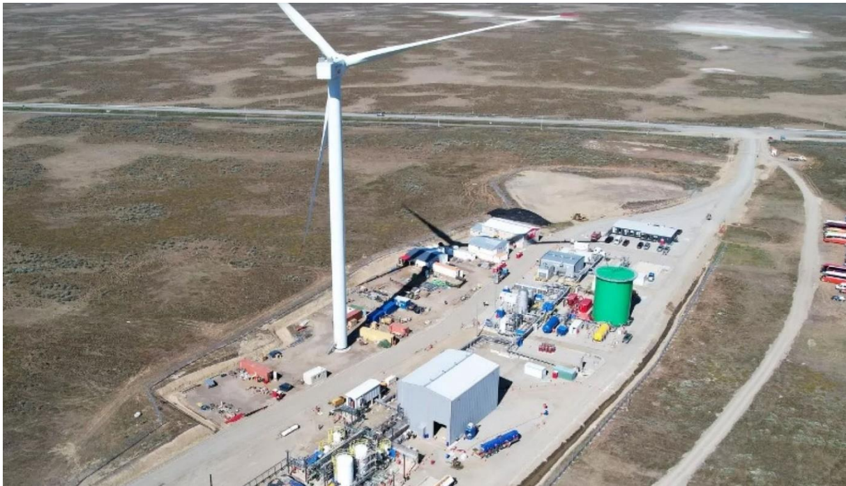
Haru Oni Demonstration Plant, a synthetic fuel plant that began operations in Punta Arenas, Chile. Source: HIF GLOBAL.
